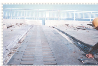
the drawing of SF type comb Expansion Joints.
