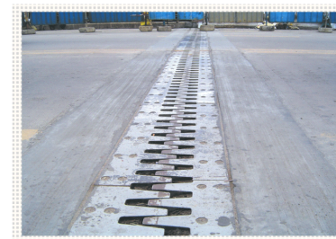
ZSF Expansion Joint under installation
