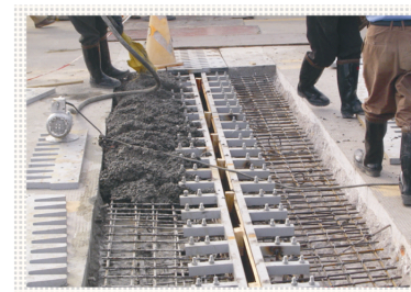
ZSF Expansion Joint under installation
